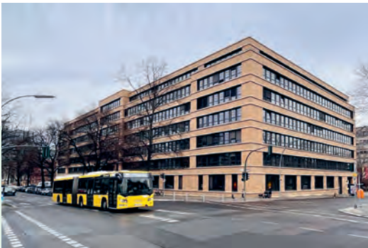
The TU Berlin's MAR building, home to SCIOI's headquarters.
